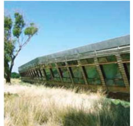
**The Outward sloping windows maximise lighting and act as solar controllers. The exposed rough sawn timber imitates coastal architecture where the building faces Swan Bay.**
