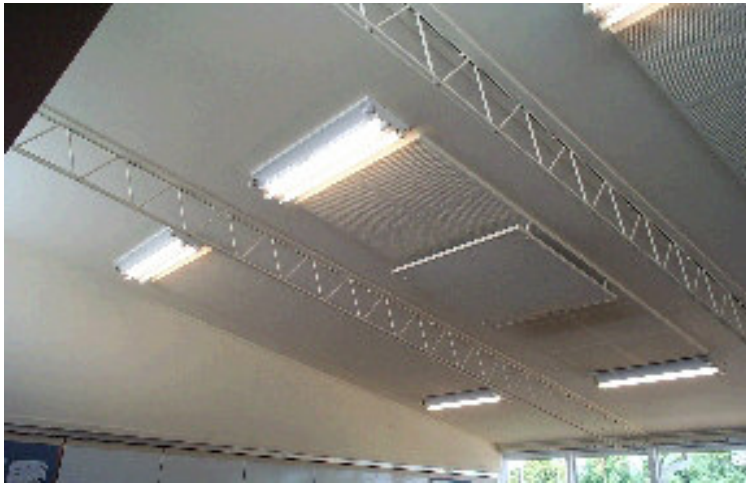
Figure 2: One of the classrooms after delamping. In each section, 6 fluorescent tubes were replaced with 3 triphosphor tubes. (Note: These rooms have excellent natural lighting and are never used at night.)
